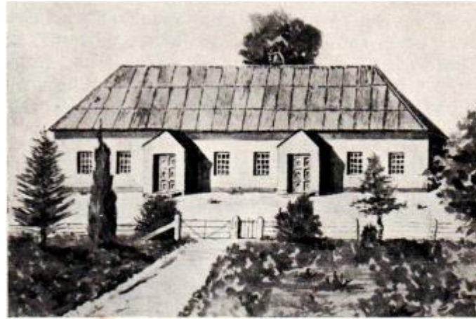
First Langmeil Church, facing east. Dedicated December 26th, 1846. Demolished 1888. (Note bell hung in gum tree behind church.)
